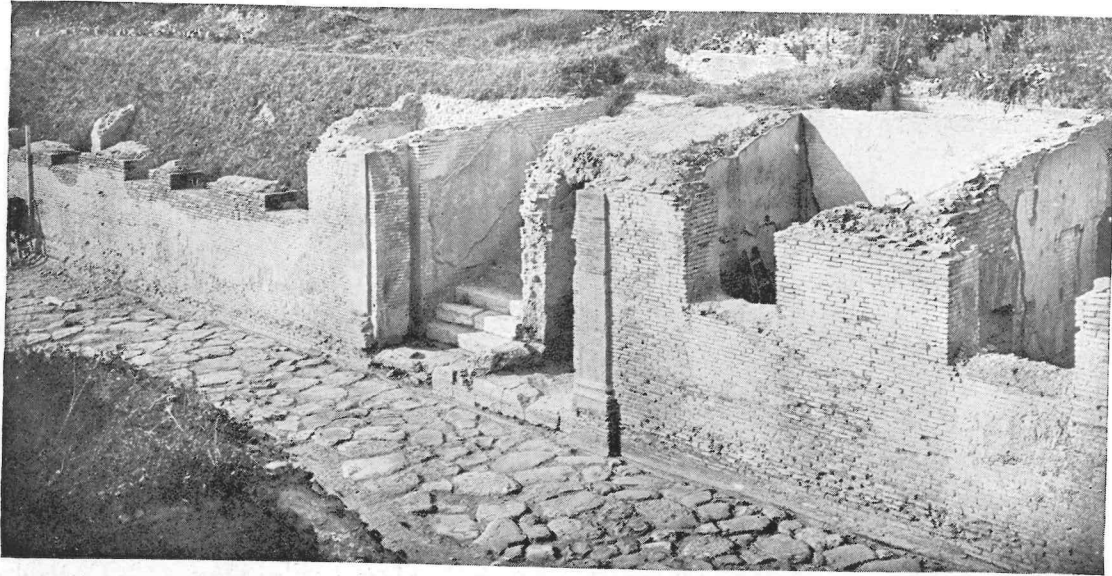
An apartment house at Ostia with a marble stairway. Inside are preserved a great many interesting pictures.
