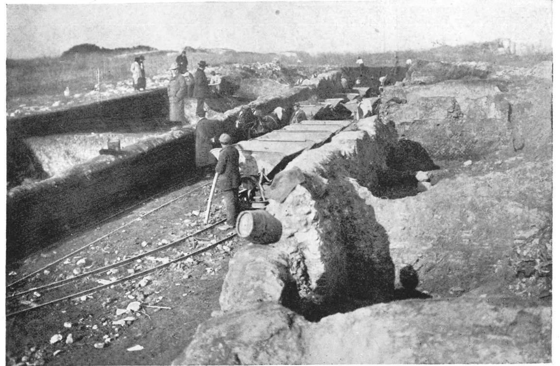
Excavating Ostia. The earth removed from the ruins is carried off on a Decanville railroad and dumped into the Tiber.
