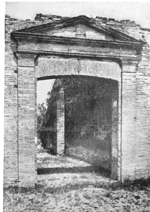
Entrance door of the offices of the Grain Measurers, one of the workmen's associations of Ostia. This is a typical example of the architectural decoration of buildings at Ostia constructed entirely of brick.
